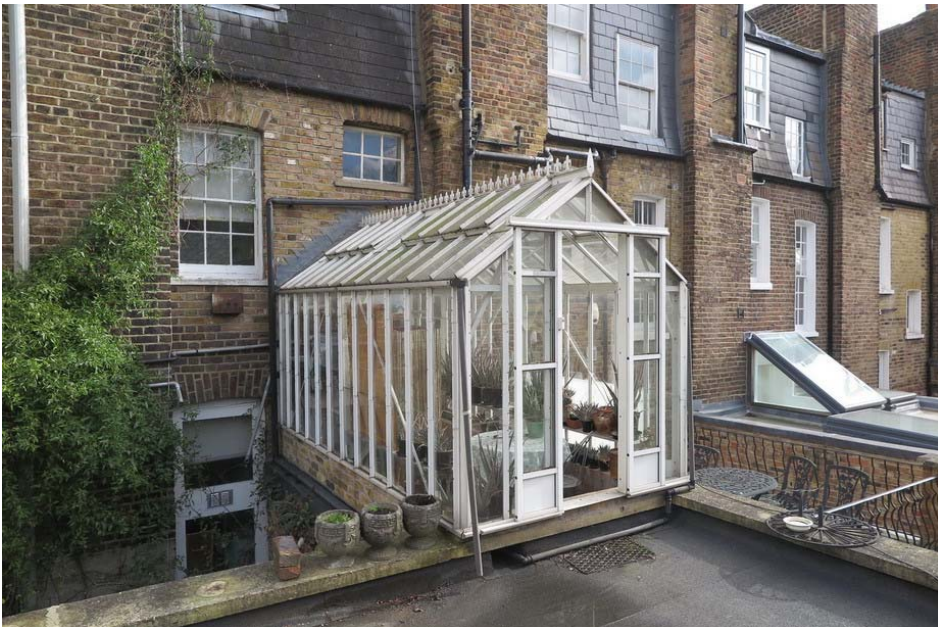
Rear view showing later addition of glass house and rear extension
