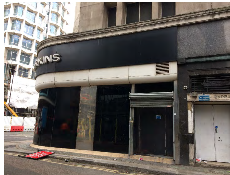
Plate 10: Bainbridge Street frontage
