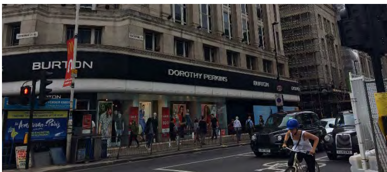
Plate 9: Modern shopfront with windows blocked by shop fittings and displays
