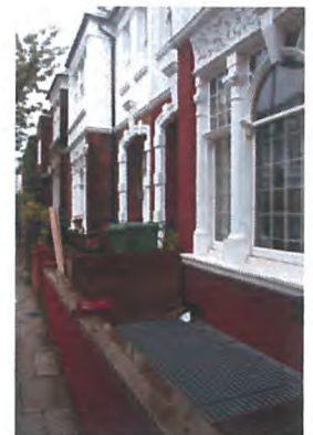
Photo 5: view of the front area of no. 43 Howitt Road, showing the white steel grille above an existing lightwell serving basement windows. no. 41 is to the left.
