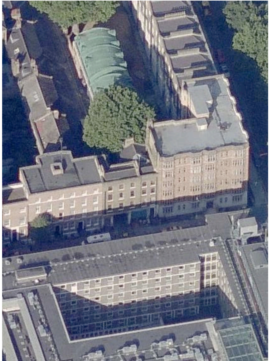
Oblique aerial view from the east
