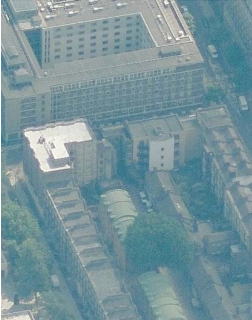
Oblique aerial view from the west
