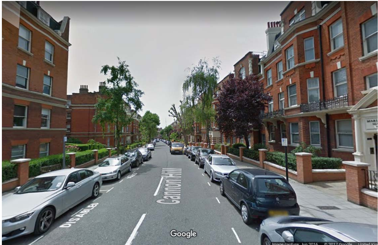
1 View of Marlborough Mansions on Cannon Hill
