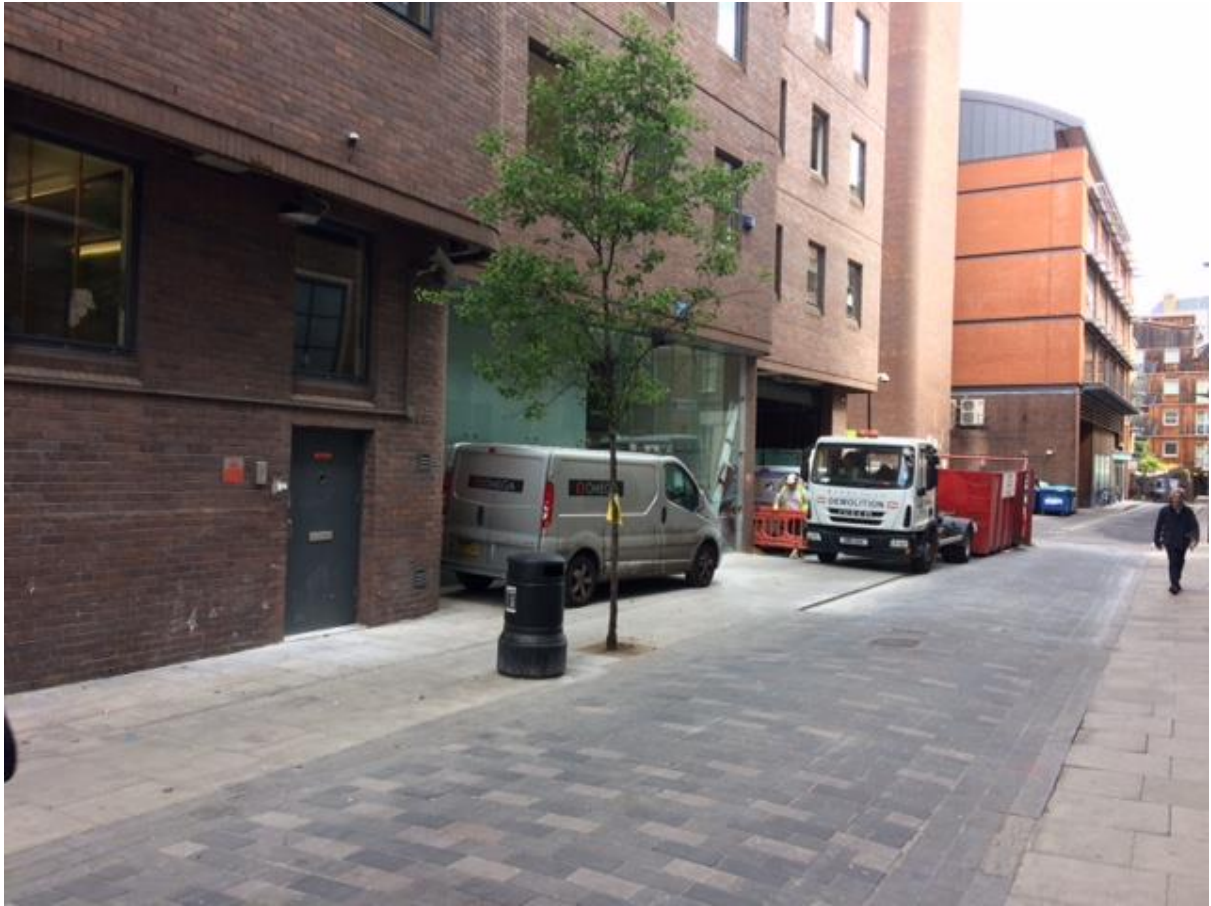
Photo 4 South Elevation – taken from Stukeley Street (showing ground floor façade)
