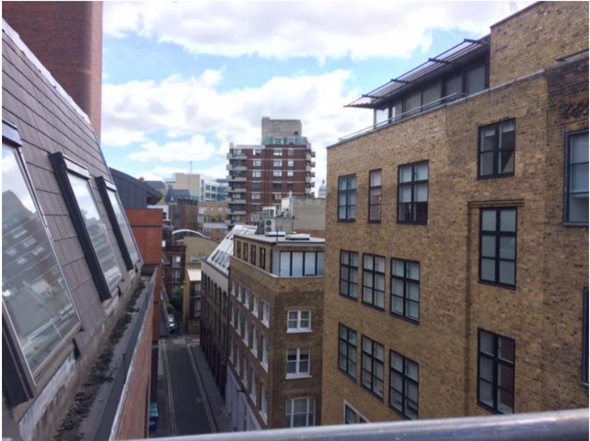
Photo 6 - Existing Roof Extension Looking East (Also Showing Roof Extensions on Buildings to the South)
