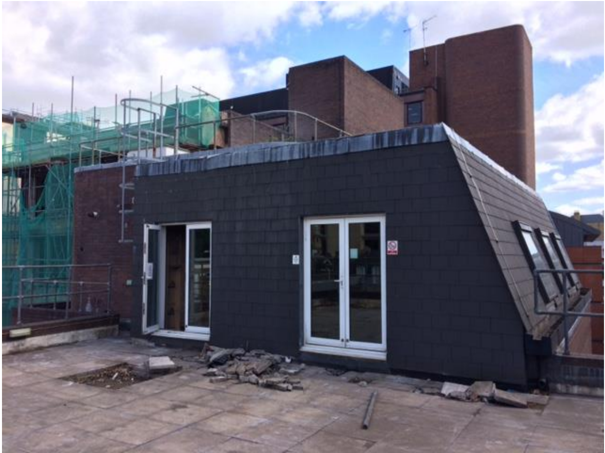
Photo 5 Existing Mansard Roof Extension from Roof Terrace
