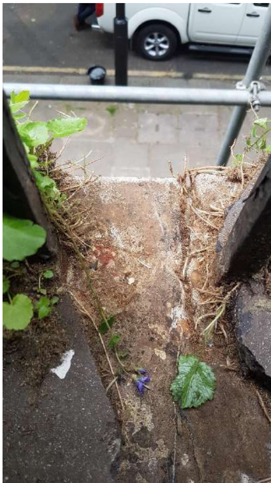
Eastern slab at edge.
