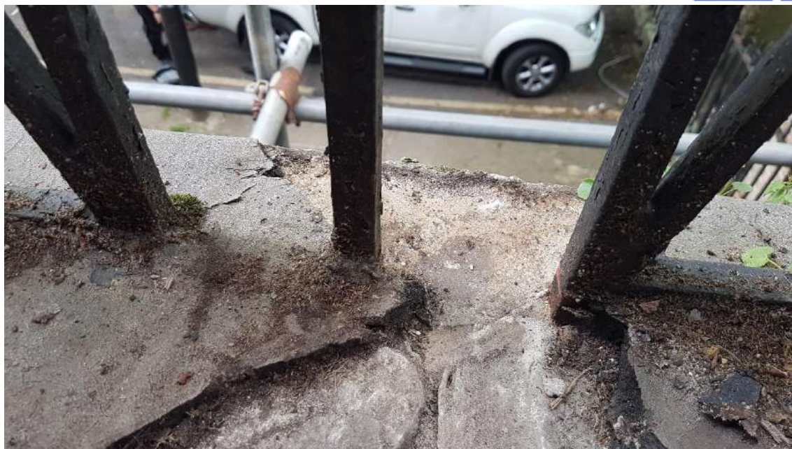
Western slab at edge.
