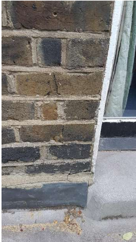
Right hand window, left reveal
