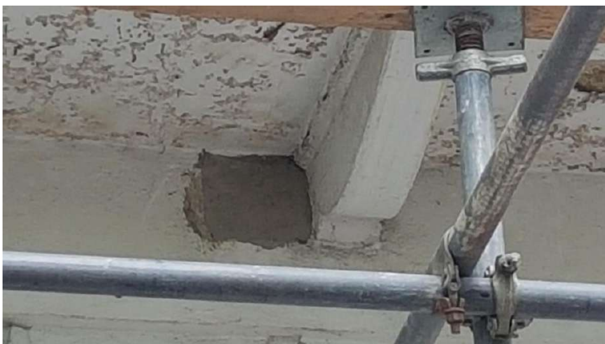
View showing the repair
