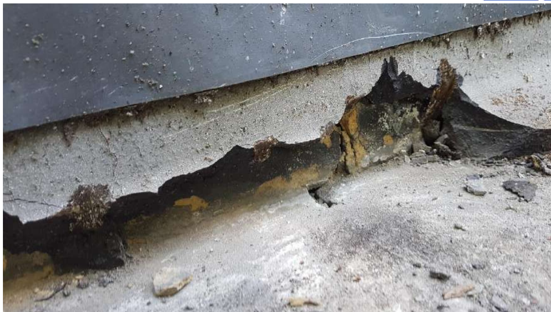
Western end with asphalt removed up to wall.
