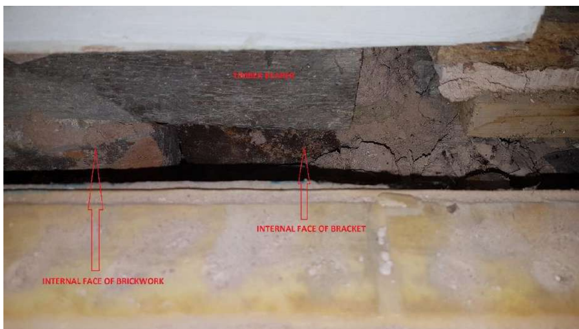
View of inner face of brickwork and rear of bracket.
