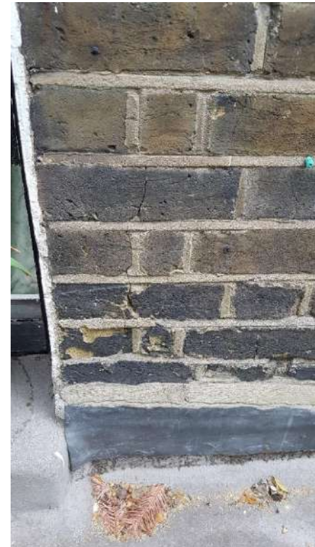
Centre window, right reveal
