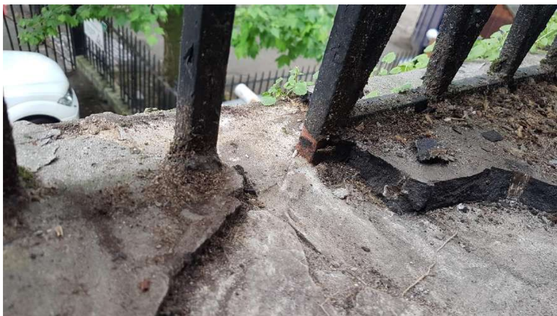
Western slab at edge.
