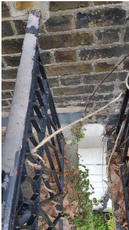
Vegetation on edge of balcony
