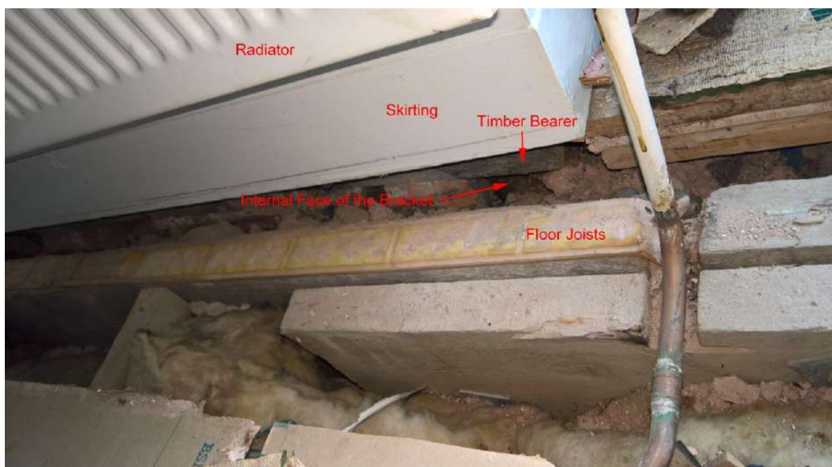
View of inner face of brickwork and rear of bracket.
