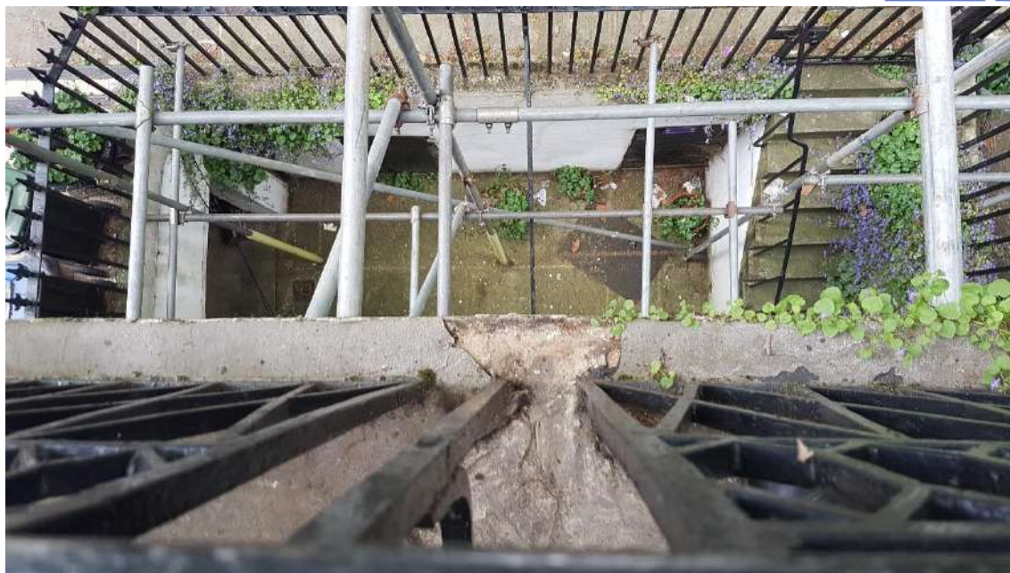
Western slab at edge.
