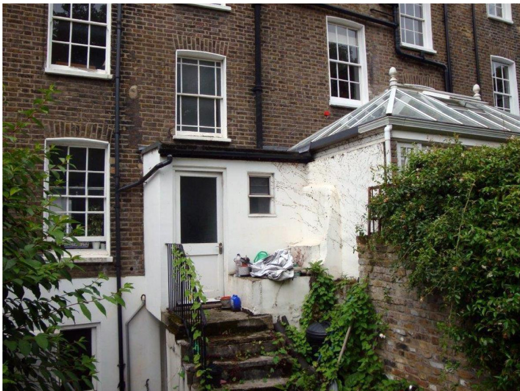
The western elevation is the back of the building.
