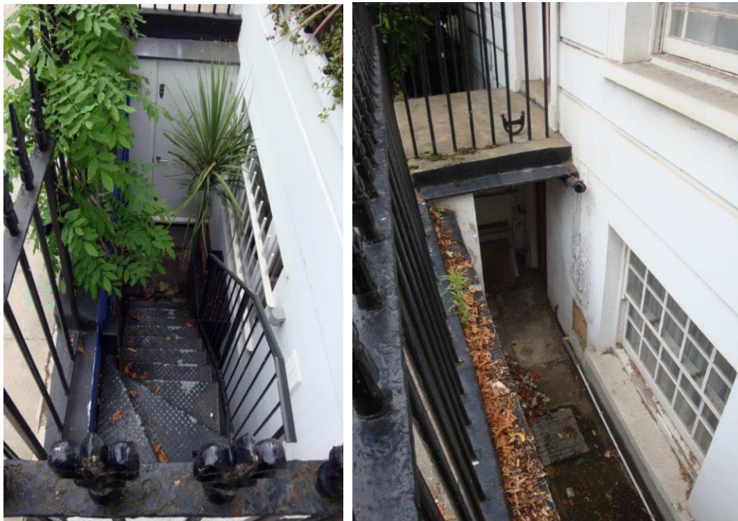
A typical staircase down into a near identical light-well to that of No94 (shown right).
