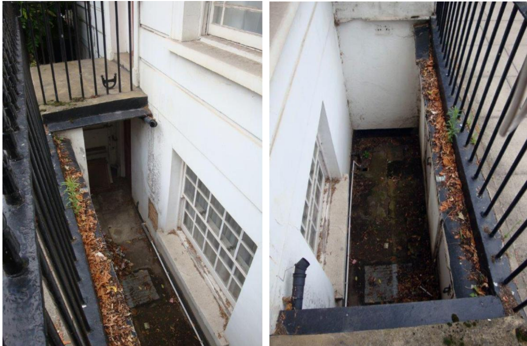
Looking N then S into the lightwell.
