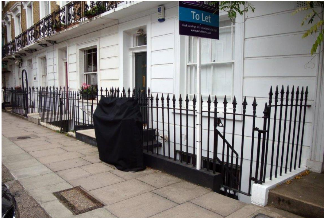
A typical staircase to near identical buildings.
