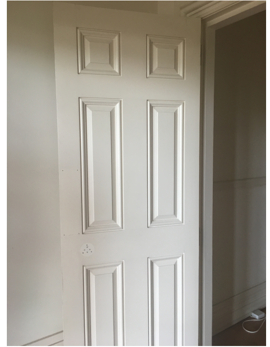
Existing non original door opening
