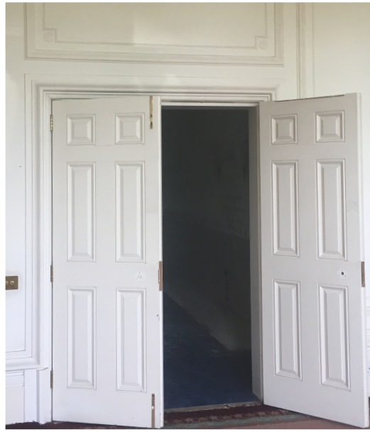
Existing doors to be replaced by new hardwood doors
