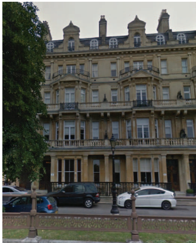
Fig 3 No 5 External View - Google Maps
