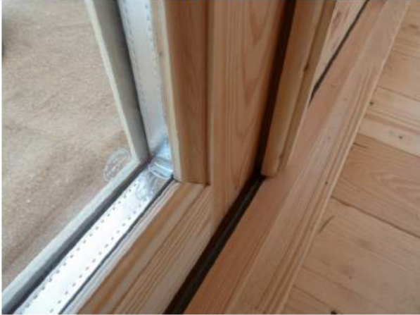
Examples of standard double-glazing (24mm)
