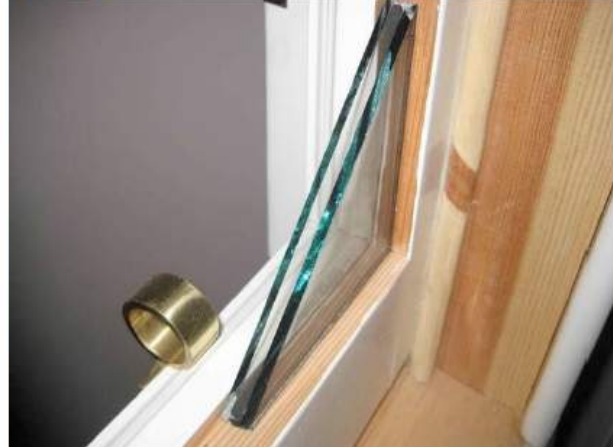
Example of slimline double-glazing (12mm)
