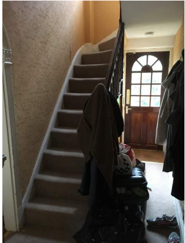
Original staircase to be retained
