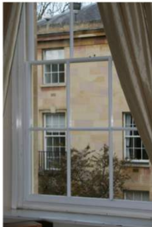
Internal View - N.B. 'traditional' simplicity, visibility of glazing spacer.
