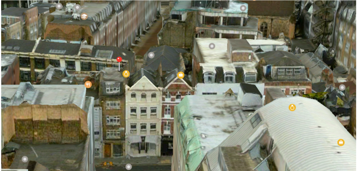
Figure 4 – Greville Street roof profile, as viewed from Kirby Street
