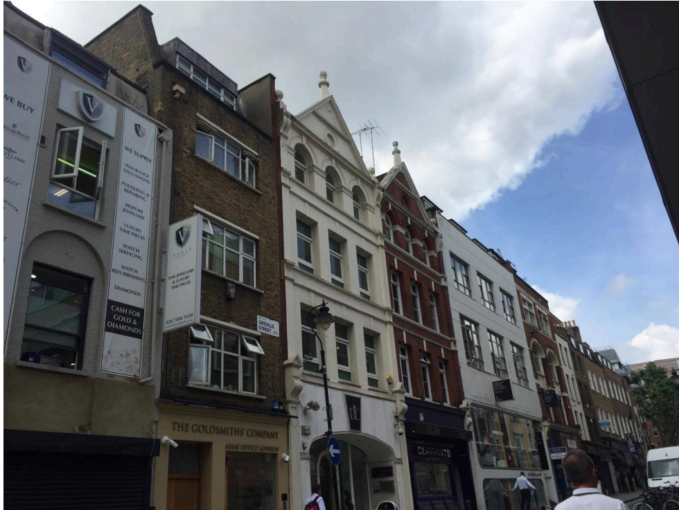
Figure 2 – Site and location context as viewed from Greville Street
