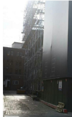
ONGOING WORKS AT NOS. 3-7 BAYHAM STREET (APPLICATION SITE IN BACKGROUND)
