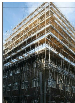
SITE UNDER CONSTRUCTION VIEWED FROM SOUTH WEST OF BAYHAM PLACE
