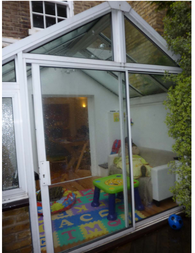
Picture 1a:Existing conservatory
