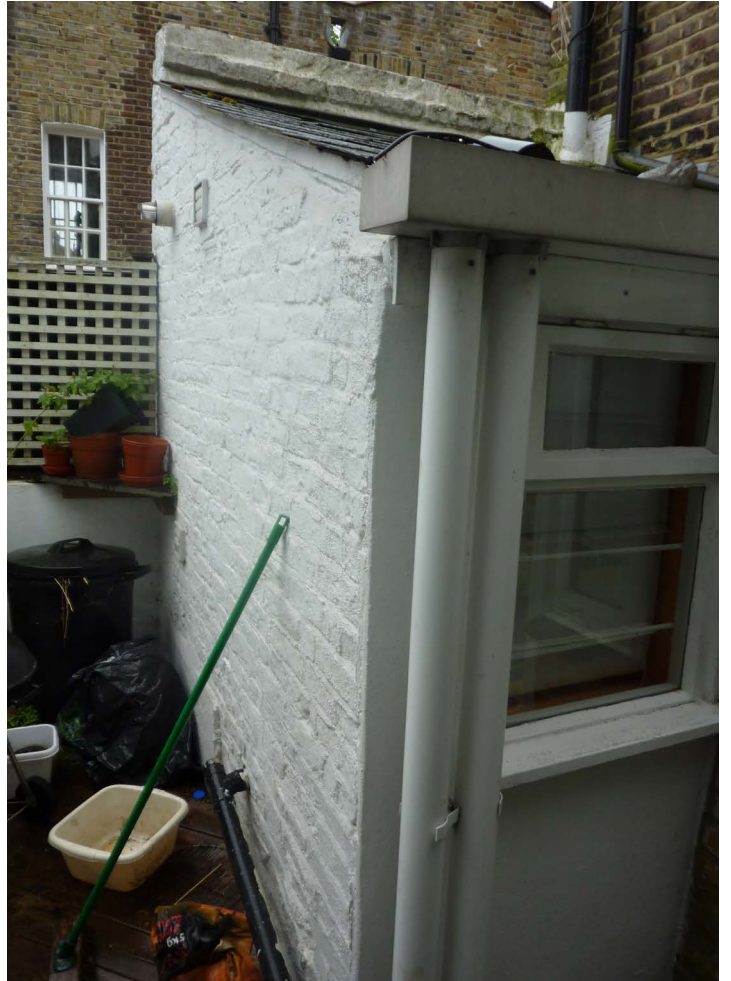
Picture 1b: Existing utility room
