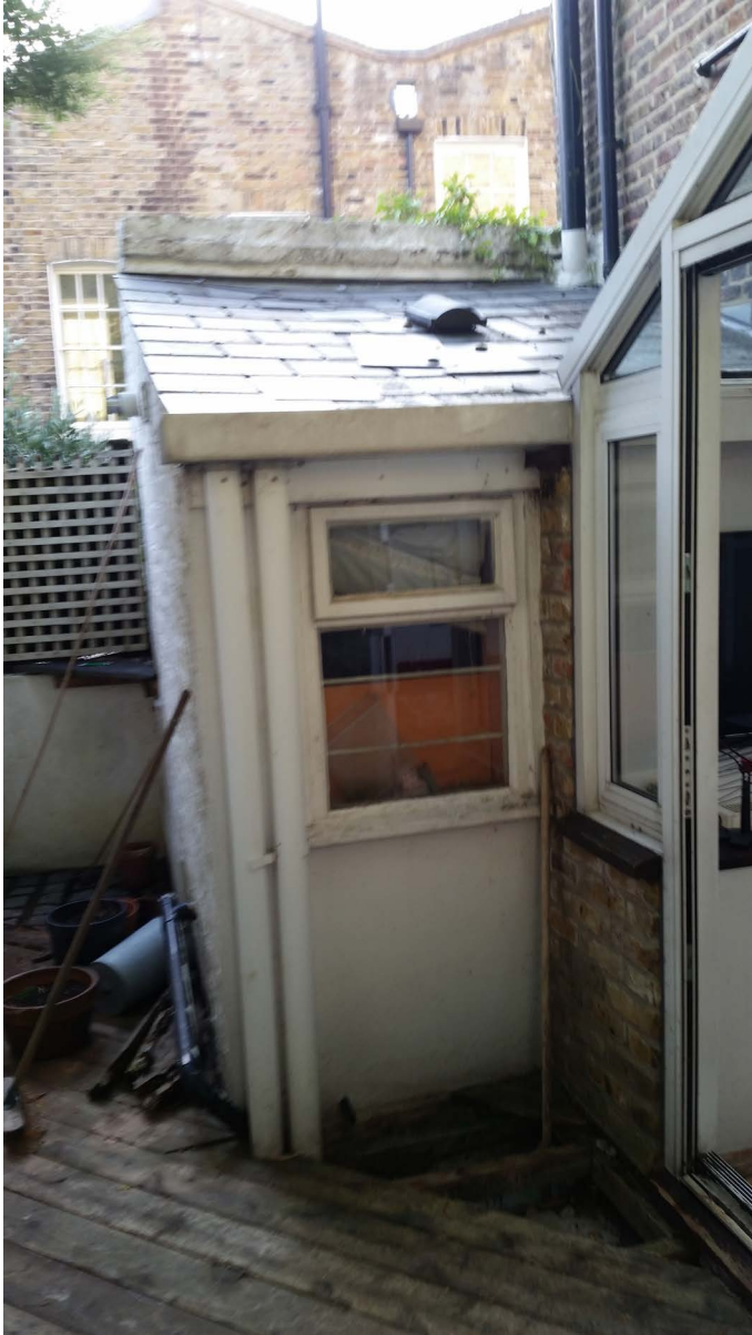
Picture 1b: Existing utility room
