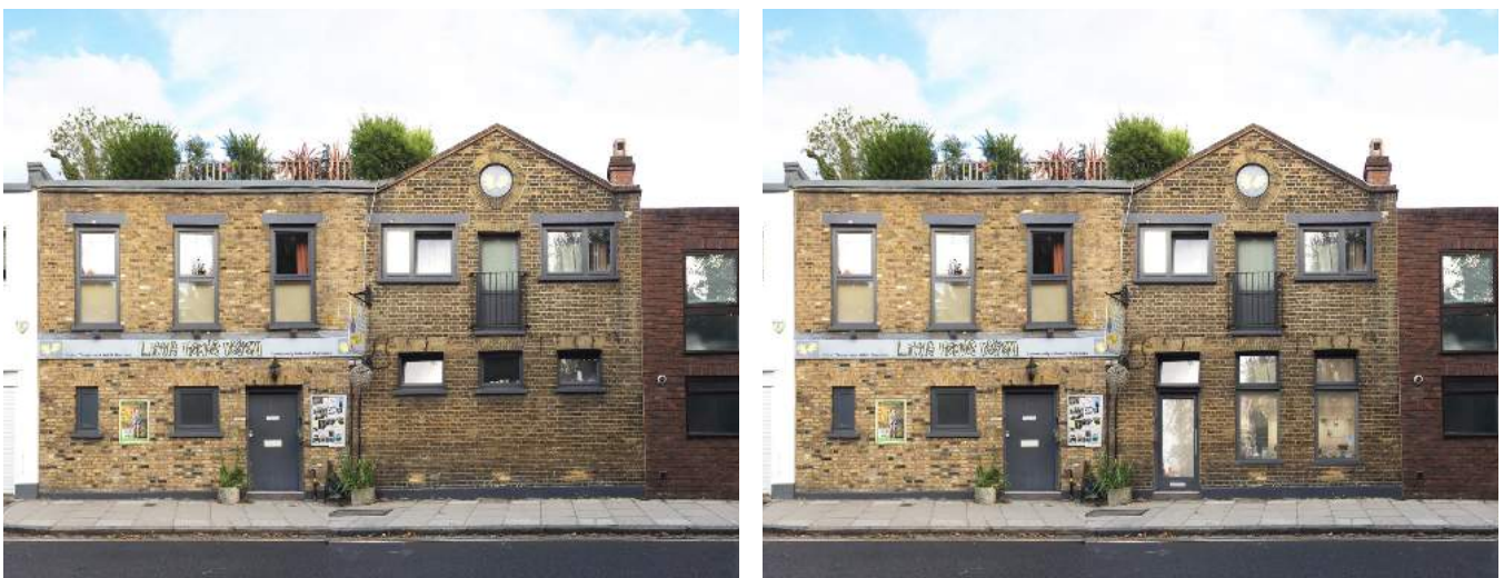
Existing and proposed views towards 67 Belsize Lane showing the integration of the existing window openings and brick lintels in the new arrangement of windows and entrance door, and the positive impact of the active street frontage.
