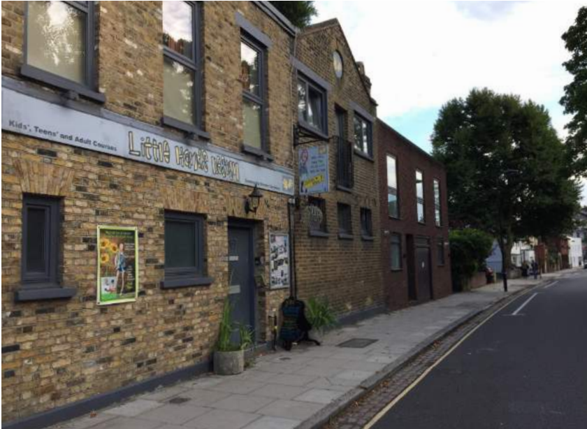
Existing street elevation to 67 Belsize Lane looking south towards the neighbouring house at number 69.
