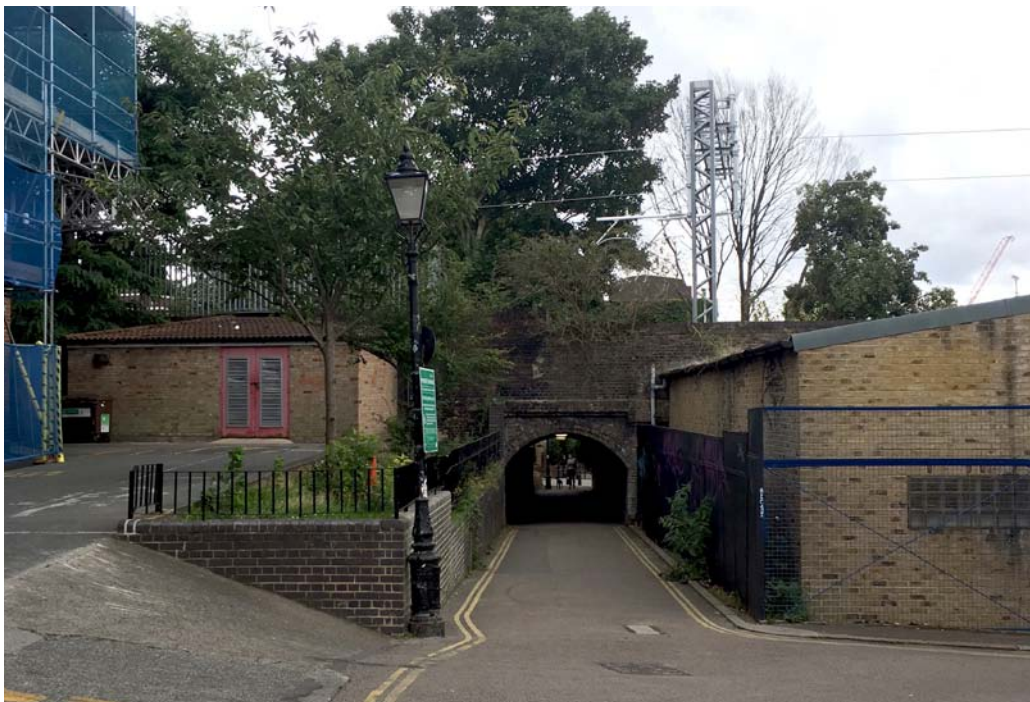
Figure 29/ Proposed view from College Lane looking south. The proposed rooftop retains a traditional silhouette as seen from College Lane and importantly remains a discrete presence with no visible light spillage or glassy reflections.
