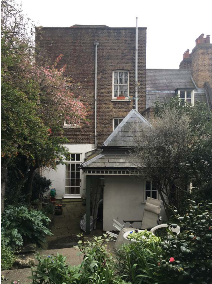
Figure 20/ Rear elevation of No. 8, 2016
