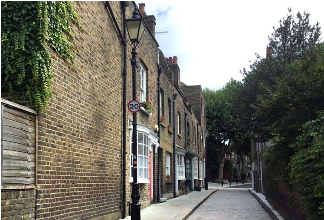
Figure 24/ Existing view of No.8 from Little Green Street looking north east.
