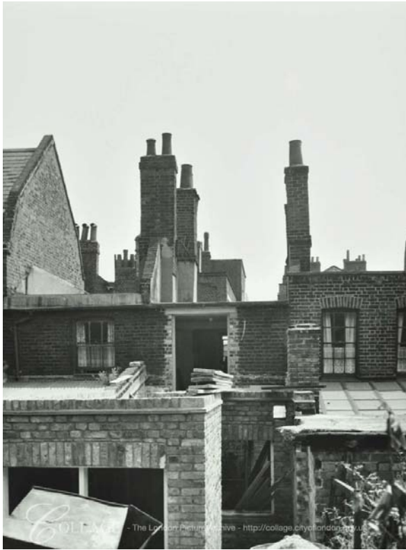
Figure 12/ Rear of No.s 4-3 Little Green Street, 1970 © London Metropolitan Archive.
