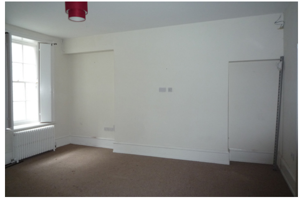
Image taken within the lower ground floor courtyard facing room prior to the 2014 application. Note the modern finishes throughout, low plasterboard ceilings and bulkhead arrangement on the far wall.
