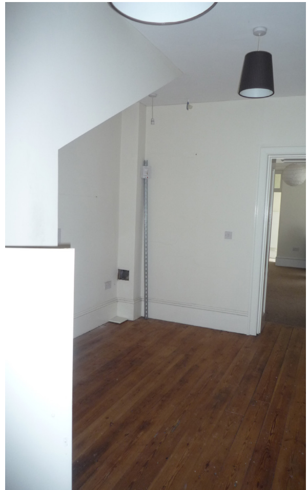
Image taken within the lower ground stair hall prior to the 2014 application. Note the modern finishes throughout, low plasterboard ceilings and the uncharacteristic open space beneath the boarded up cantilevered stone stair intended to connect the lower ground and ground floor levels.
