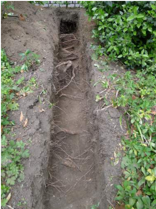
Figure 4.8d Trial pit excavation
