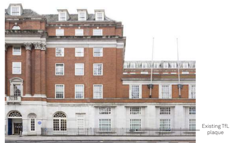
Figure 4.2f Elevation showing existing TfL plaque on BMA railings (Grade II listed building)
