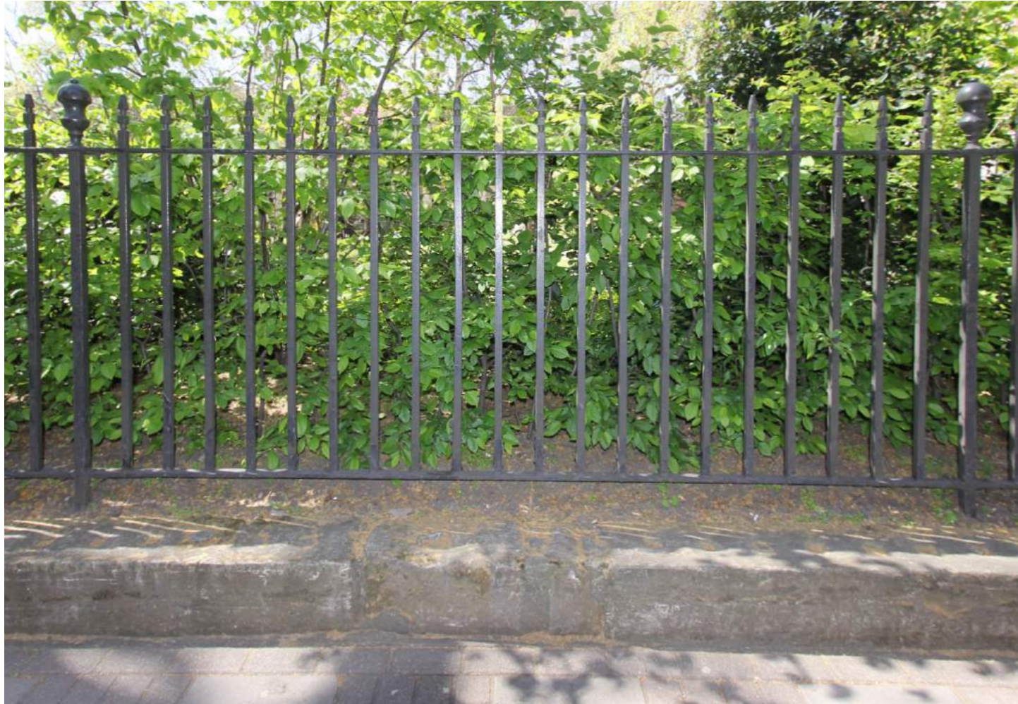
Figure 3.6a Existing railings above proposed memorial location.
