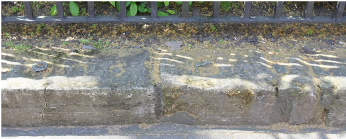
Figure 3.6b Existing Georgian kerb stone
