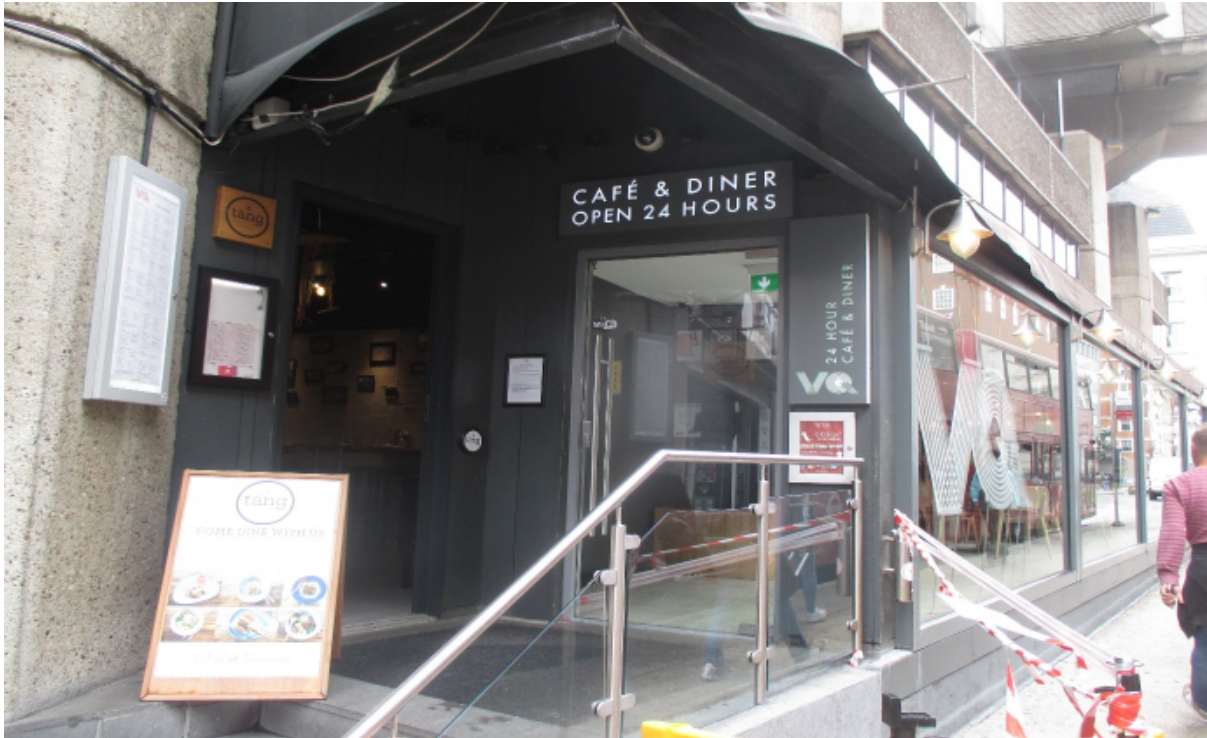
1. Photo showing NW door entrance with existing sign to be replaced.
