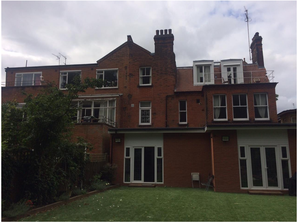
7. Rear elevation of the host property
