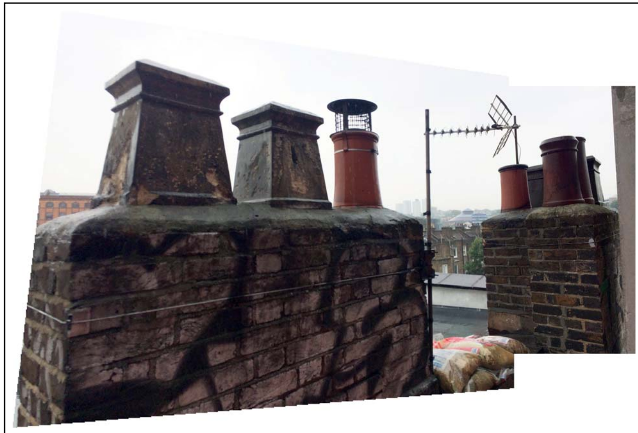
Existing condition of Chimneys
