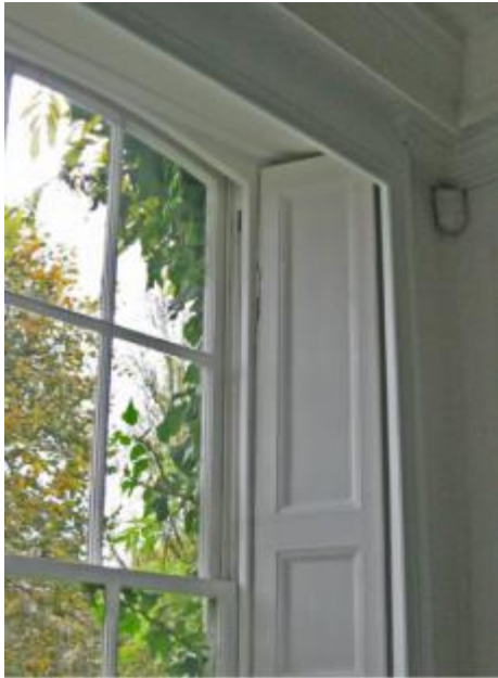
Figure 1: Examples of Internal Secondary Glazing installed in a Grade 1 listed Nash building.
