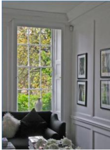
Figure 1: Examples of Internal Secondary Glazing installed in a Grade 1 listed Nash building.
