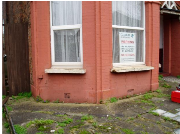
Fig. 2. Front yard with extensive hardstanding
