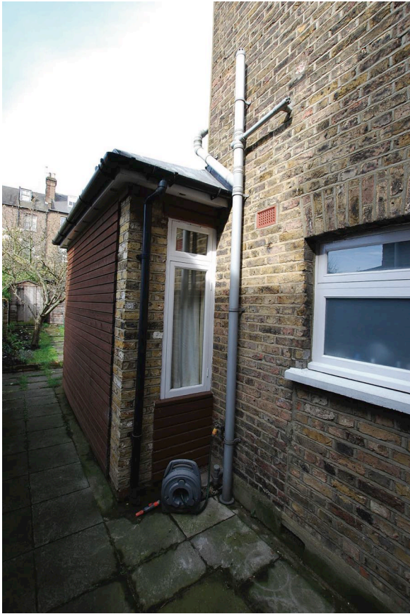
Side of Existing Extension Towards the Garden
