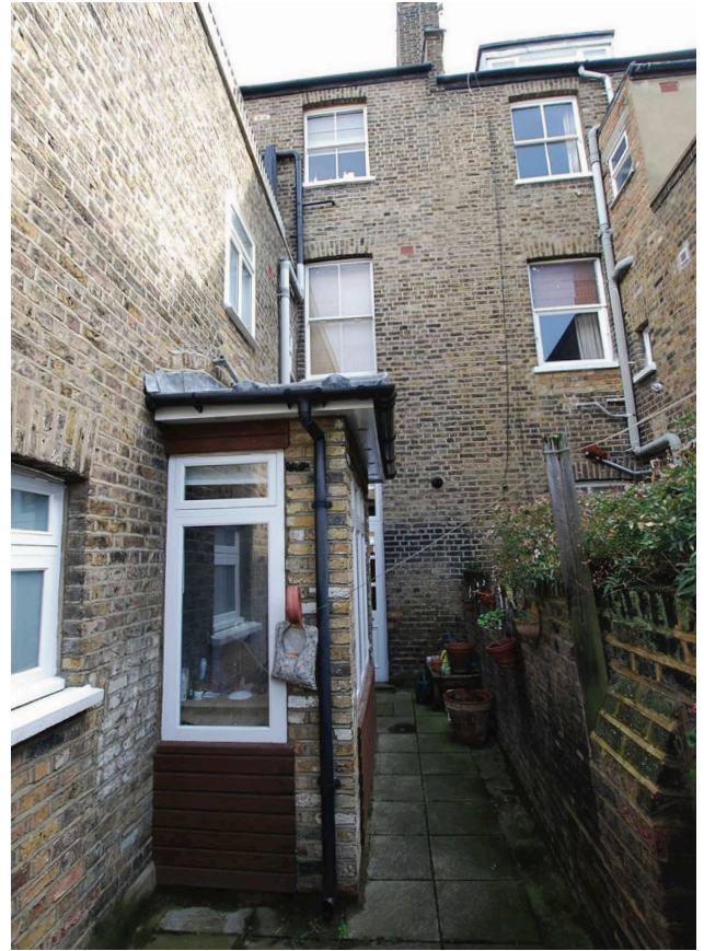
Side of Existing Extension Towards the House
