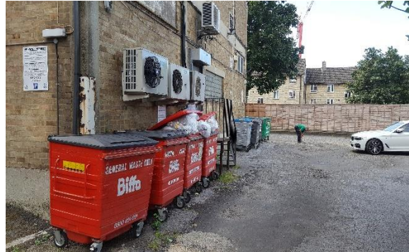
Image 2 – Existing air condensers along western elevation
