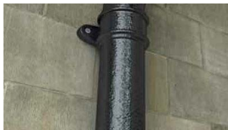
Figure 3: cast iron RWP
