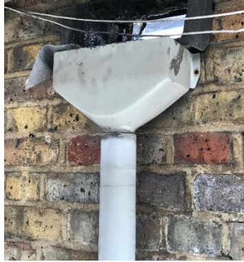
Figure 2: existing PVC rainwater pipe on Sandwich Street façade
