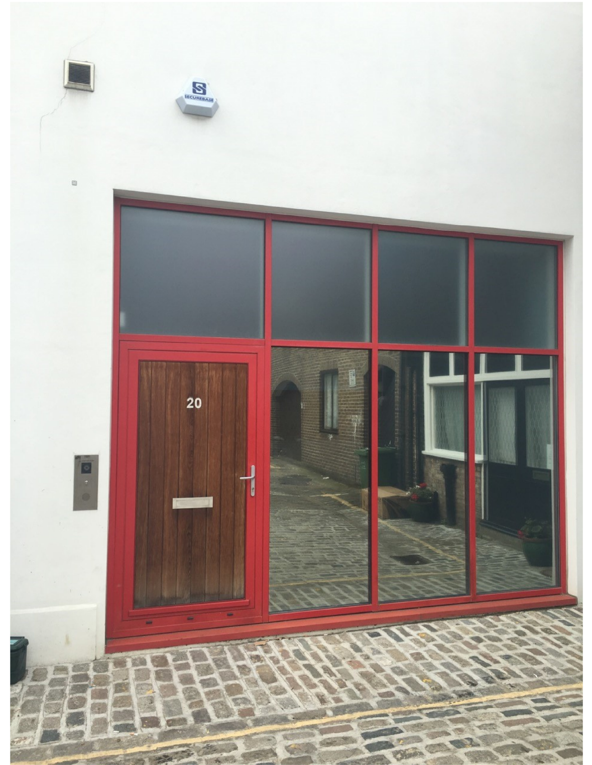
20 GRAFTON MEWS, GROUND FLOOR ENTRANCE AND WINDOWS
