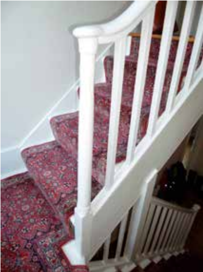
23. Main staircase showing the original balustrade and three later balusters at the top of the ground floor flight (2016), DIA
