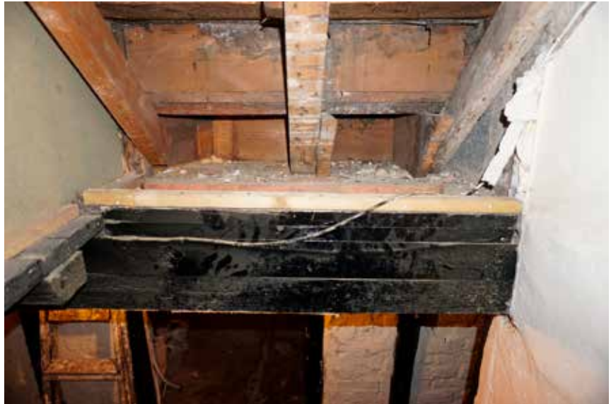
26. Original ground floor stair trimmer, now redundant due to the relocated position of the stair, (2017) DIA
