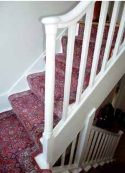
23. Main staircase showing the original balustrade and three later balusters at the top of the ground floor flight (2016), DIA
