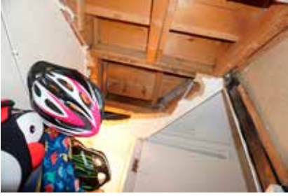
22. Late-19th century rebuilding of the ground floor staircase, the original winders can be seen at the top (2017), DIA
