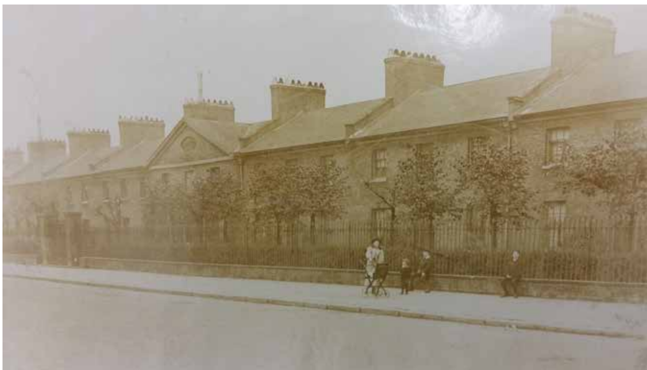
9. Late-19 th century photograph of 1-7 St Martin's Almshouses showing the original central windows at first floor level, Camden Archives
