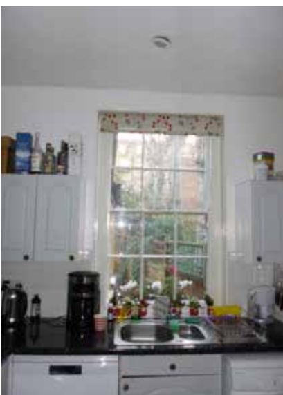
24. Original six-over-six sash in the ground floor kitchen, room G03 (2016), DIA
