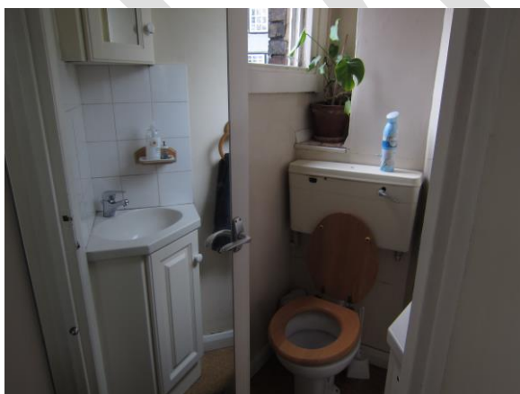
Fifth floor office wc
