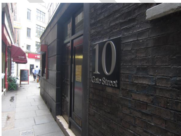
The western elevation on Little Turnstile Street (taken in a northerly direction)
