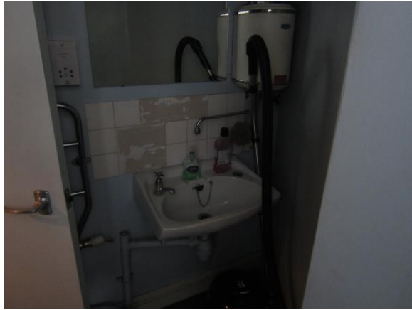
Third floor wc
