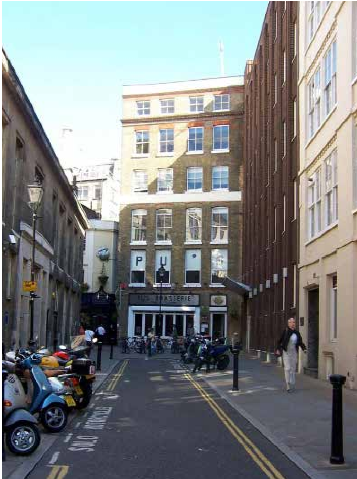
Existing south facade to Gate Street.
