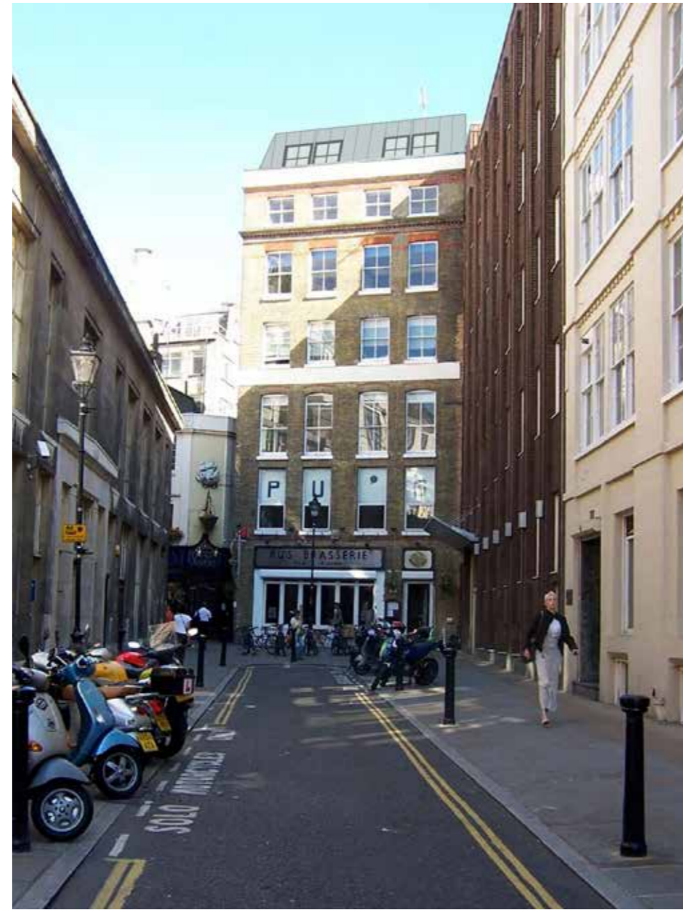
Previous view from Gate Street showing mansard roof.
