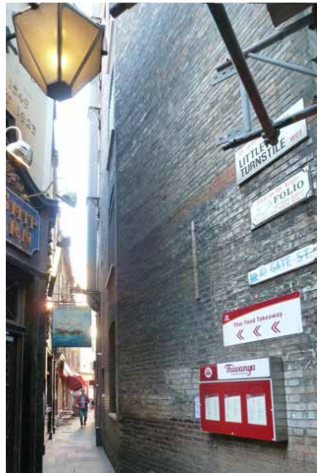
Existing Looking North along Little Turnstile Street
