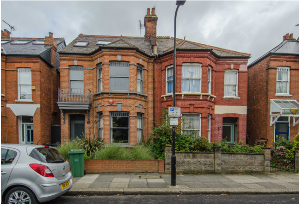
7 Richborough Road NW2 3LU South Elevation (Front )
