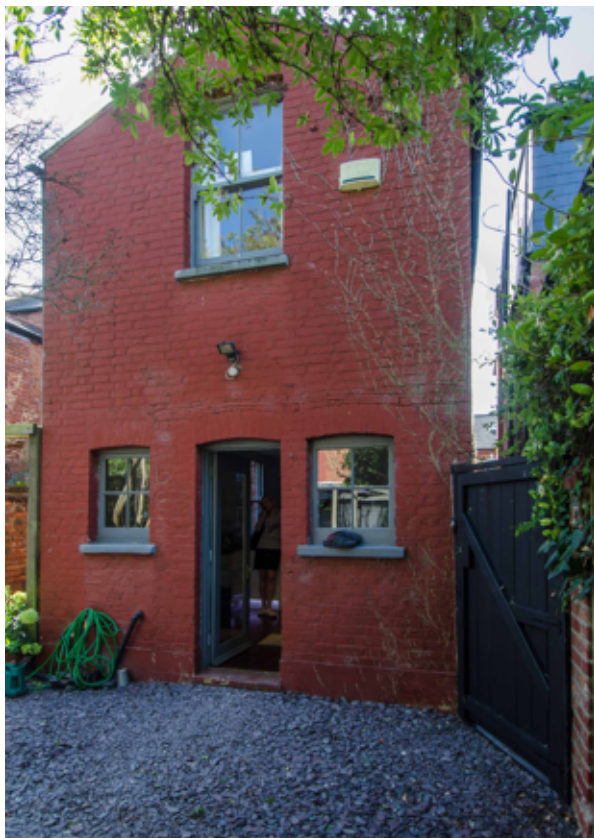
7 Richborough Road NW2 3LU North Elevation (Rear )
