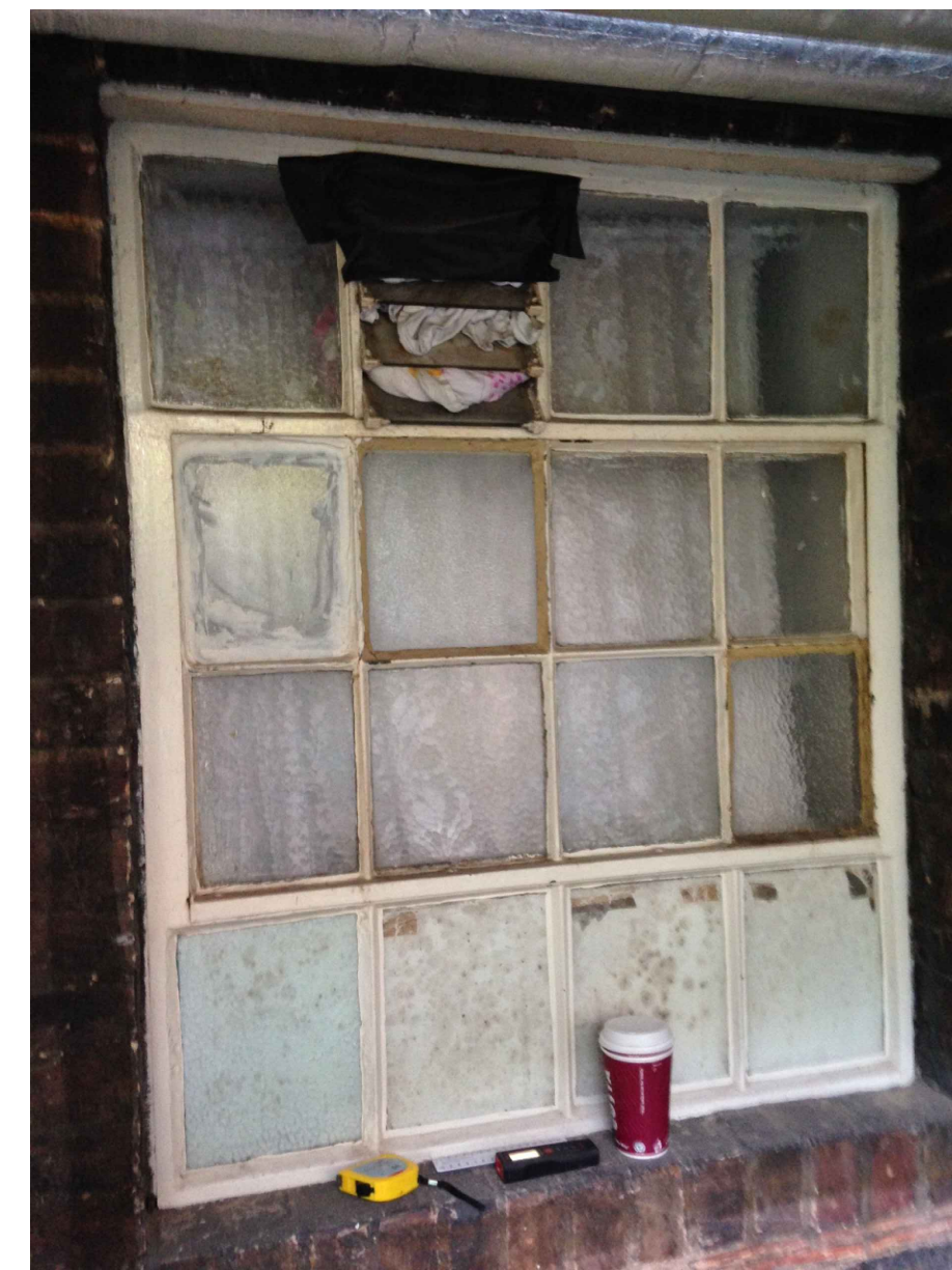
IMAGE 1 OF EXISTING WINDOWS
