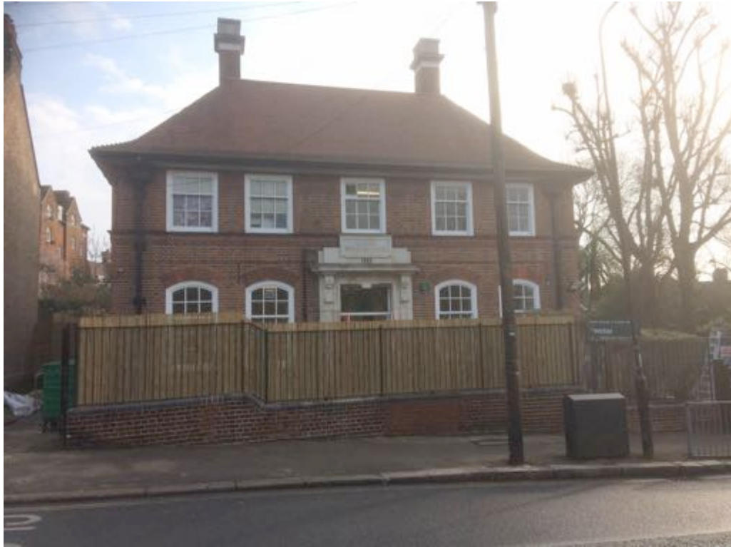
Existing elevation from Chester Road, showing bamboo screen to 2-3 year olds external play
