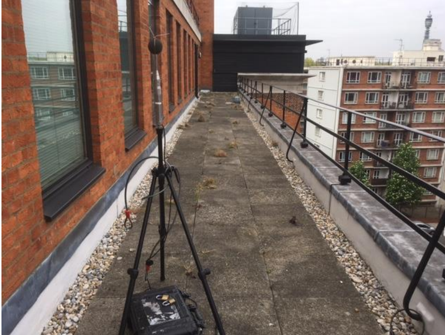
Figure 2 Photograph of unattended logger on 6th floor balcony
