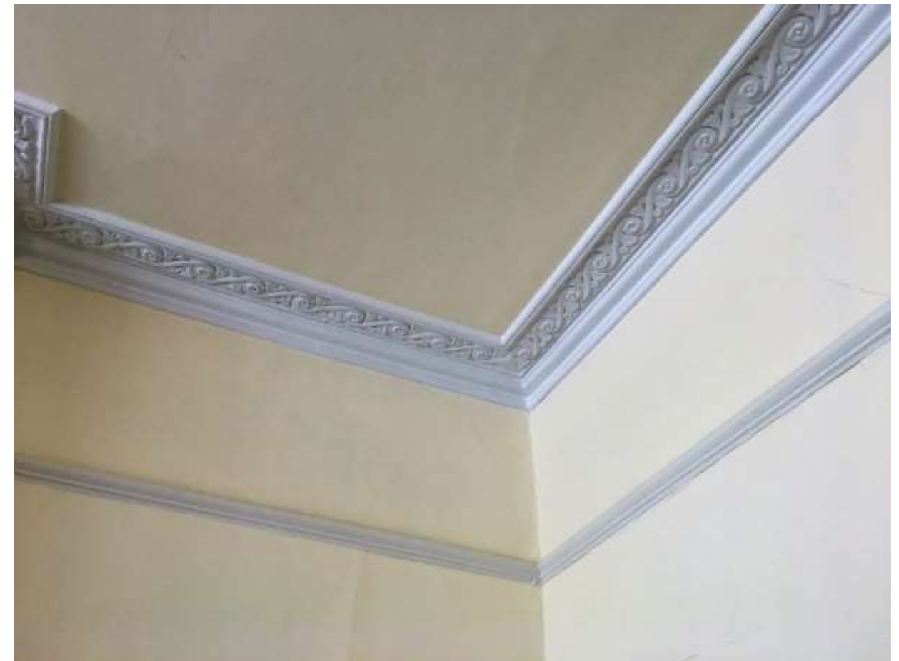
Plate 10: Ground floor cornice detail
