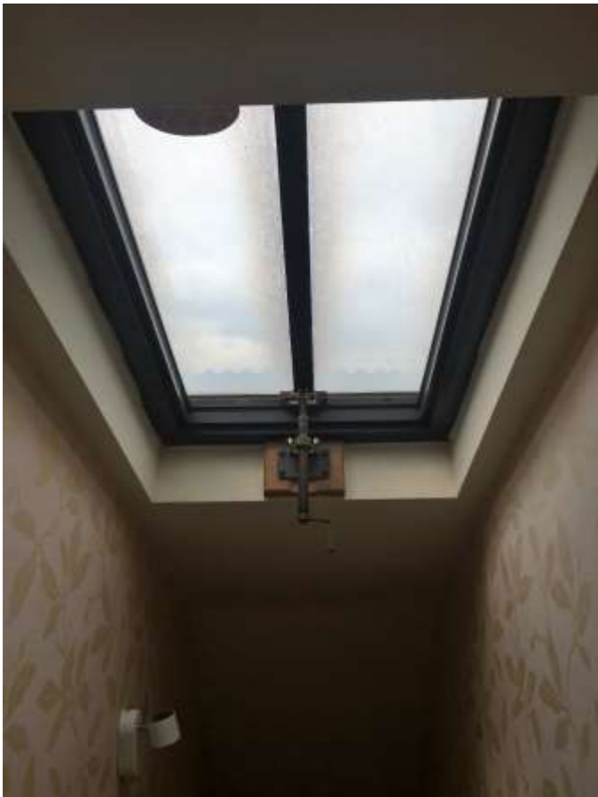
Plate 4: Later inserted roof light over staircase
