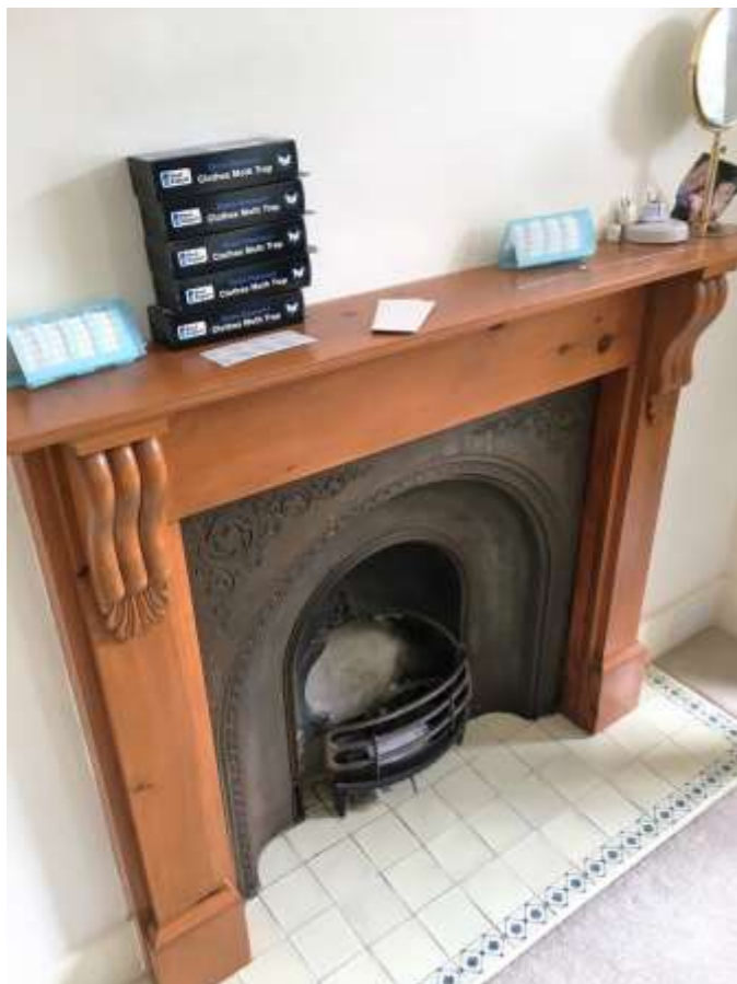
Plate 11: Historic fireplace insert and later surround at first floor
