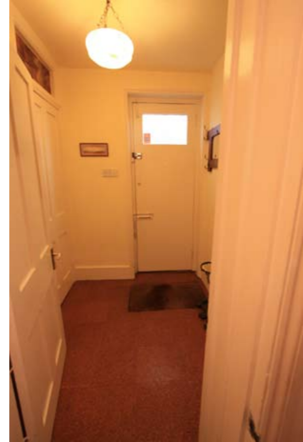
Side Entrance, also showing the double wall detail on the right of the office entrance
