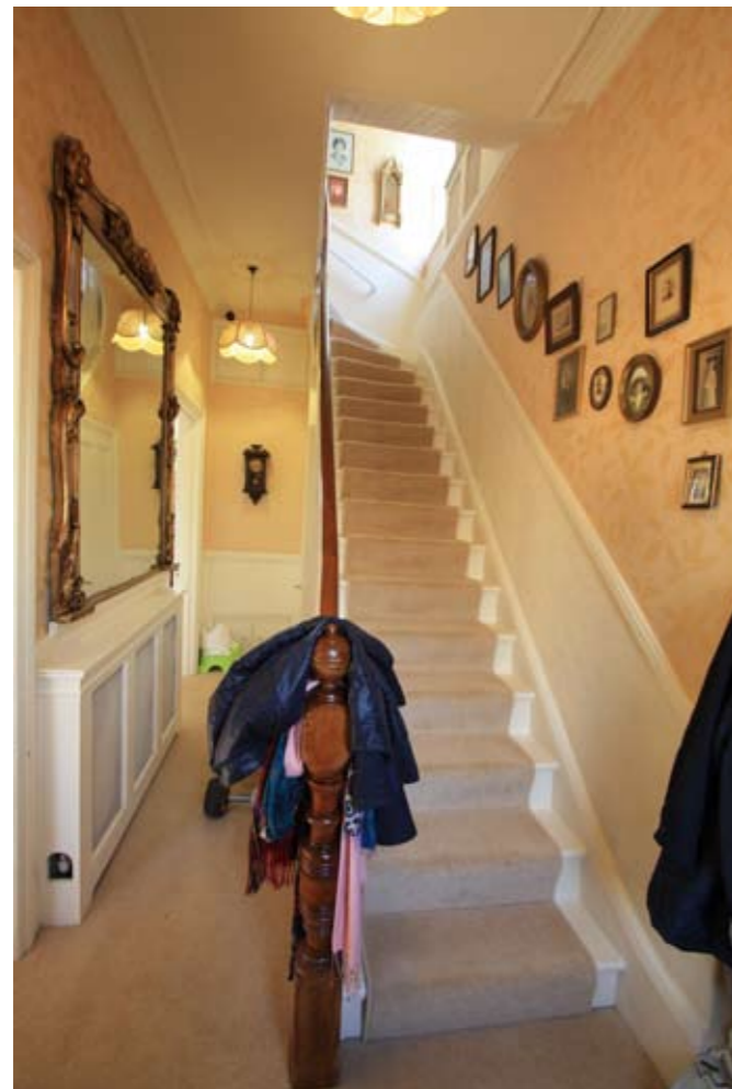
Staircase to First floor, showing the non-original newel post
