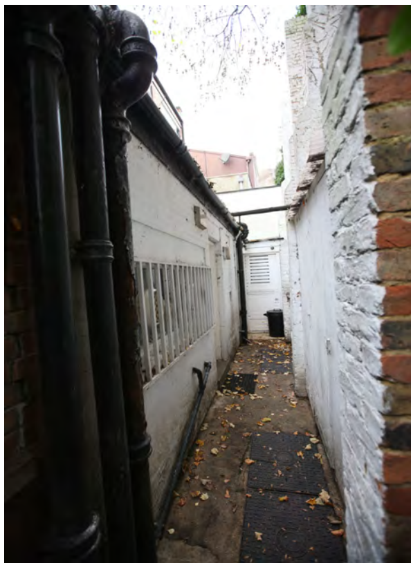
Looking towards rear of 4 Oak Hill Park Mews, London NW3 7LH
