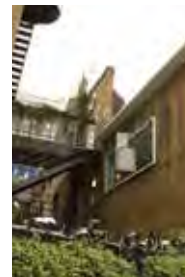
New / Old junction
