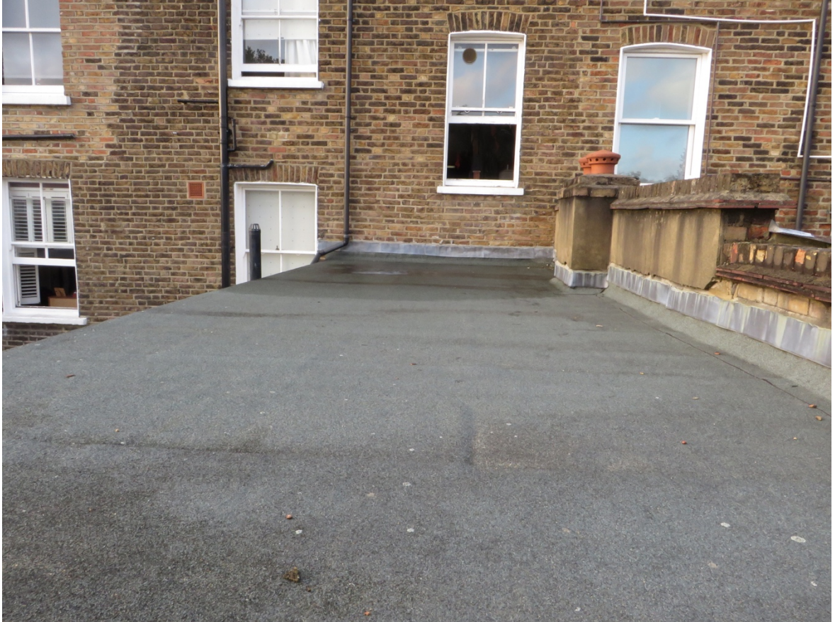
Figure 3.3: existing roof looking north towards main terrace
