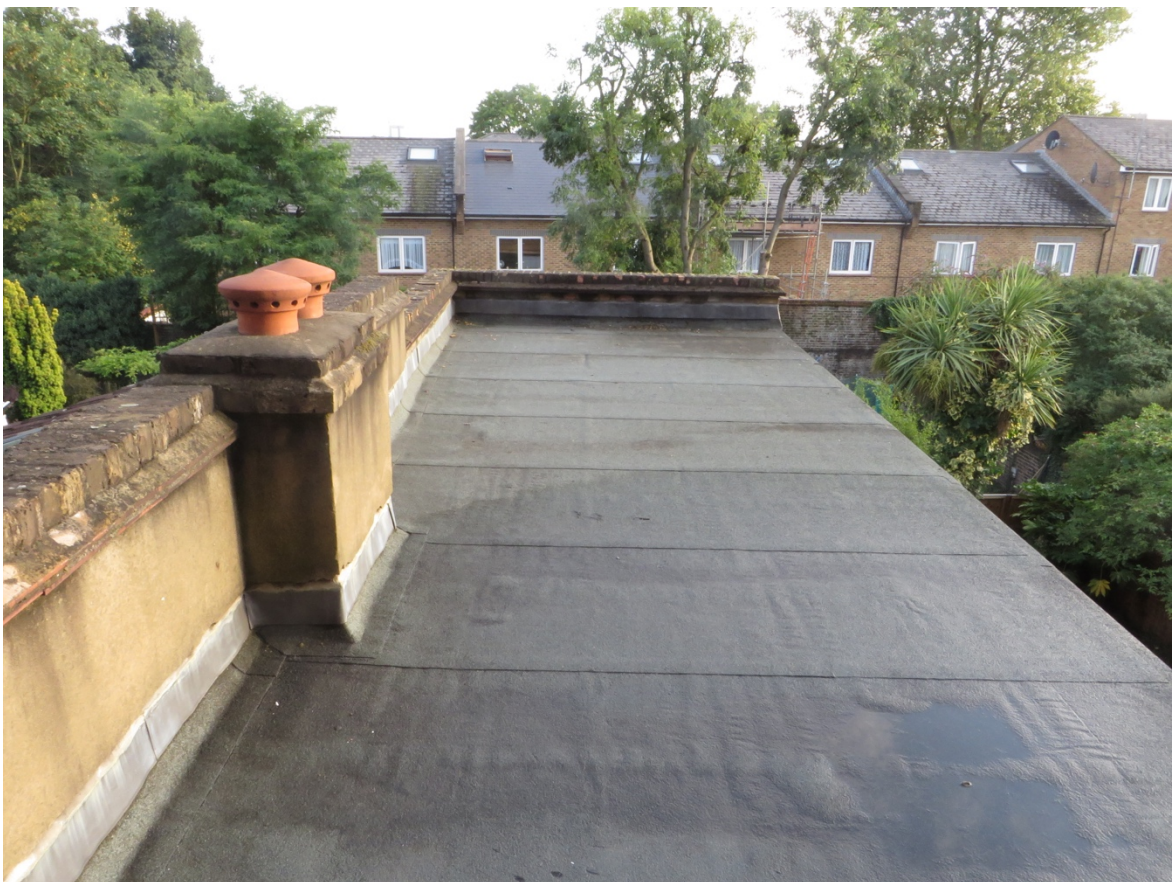
Figure 3.2: existing roof looking south from position of proposed access door
