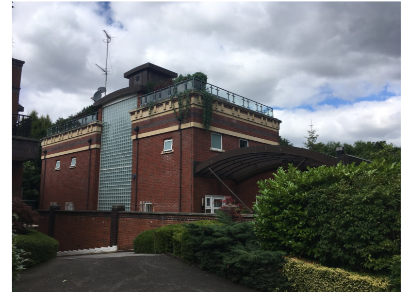
Figure 20: The site showing irregular roof form completely out of place with the rest of the conservation area.
