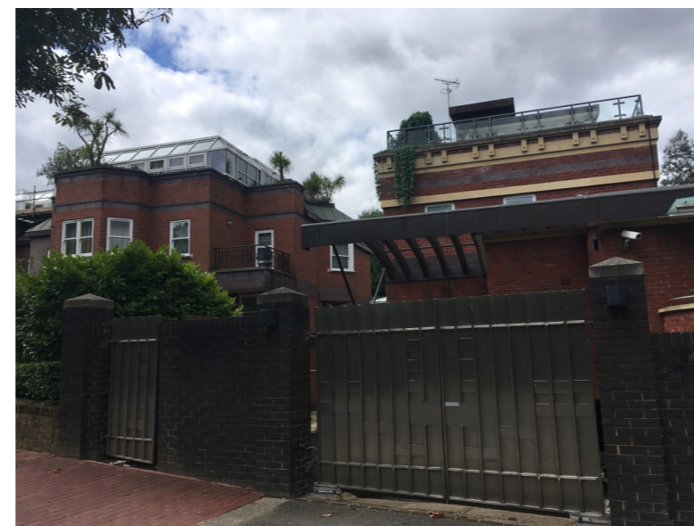
Figure 19: View of eastern elevation of house, showing No. 33 Templewood Avenue with its existing glazed roof extension and projecting canted bay.
