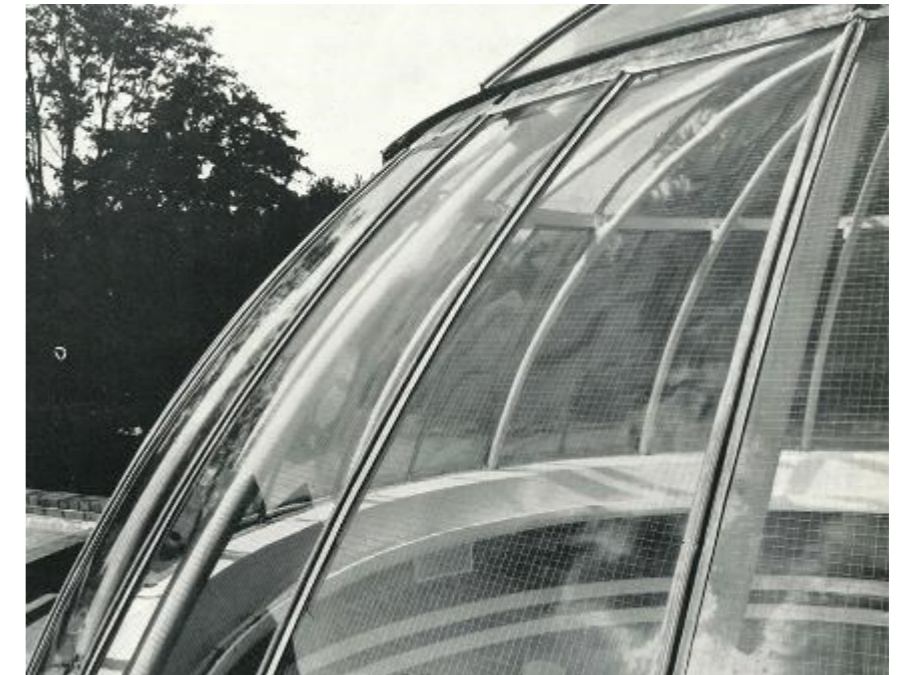
Figure 12: Historic photograph showing Georgian wire glass, now lost
