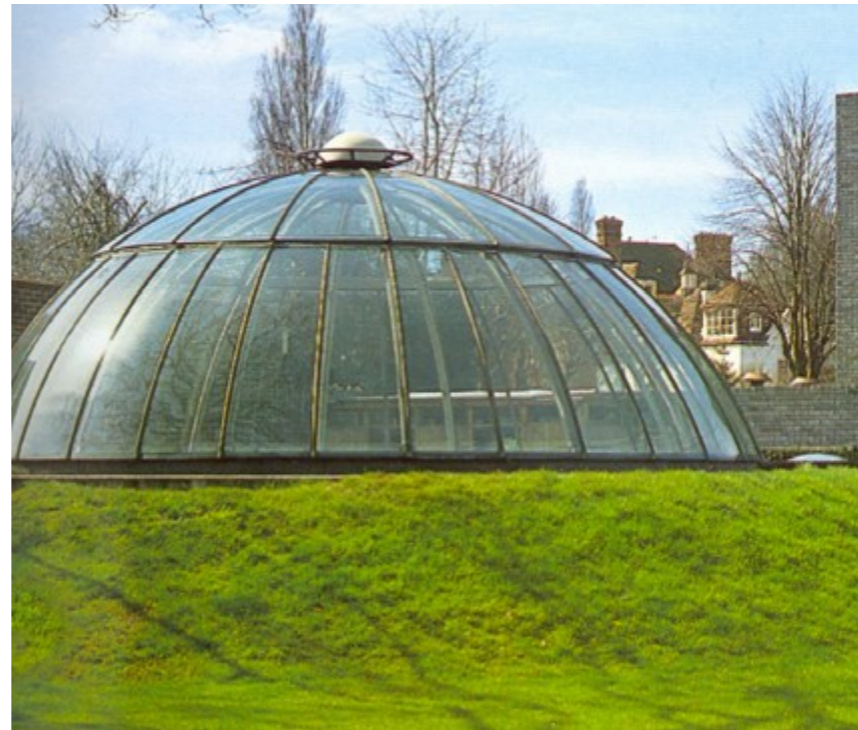
Figure 10: Early photograph showing the pool's original mound and its clear relationship with Schreiber House. Here the pool integrates seamlessly into the landscape
