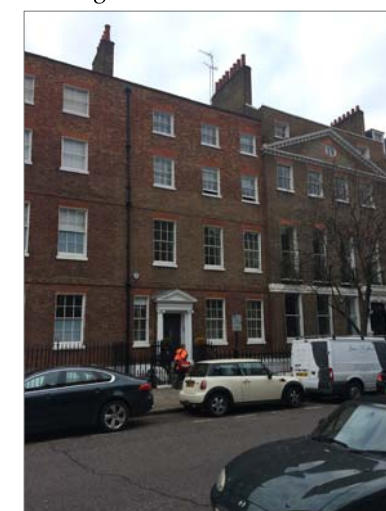
Existing windows of Front facade
