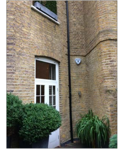
Existing windows at first, second floor Rear facade
