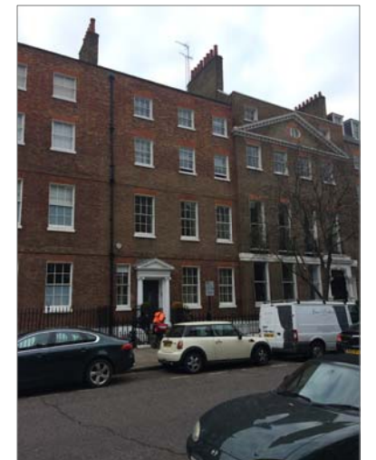
Existing windows of Front facade
