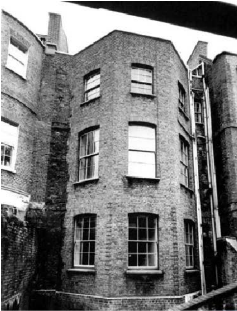
Photo from 1968 showing the rear elevation of no. 34 before the basement and third floor extensions
