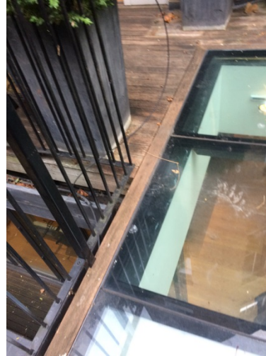
Roof Light in terrace
