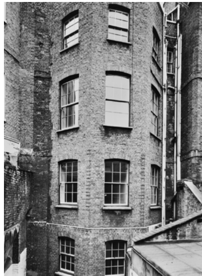
Rear elevation of 34 John Street in 1960
