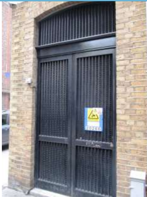
Example of Existing Louvred Door
