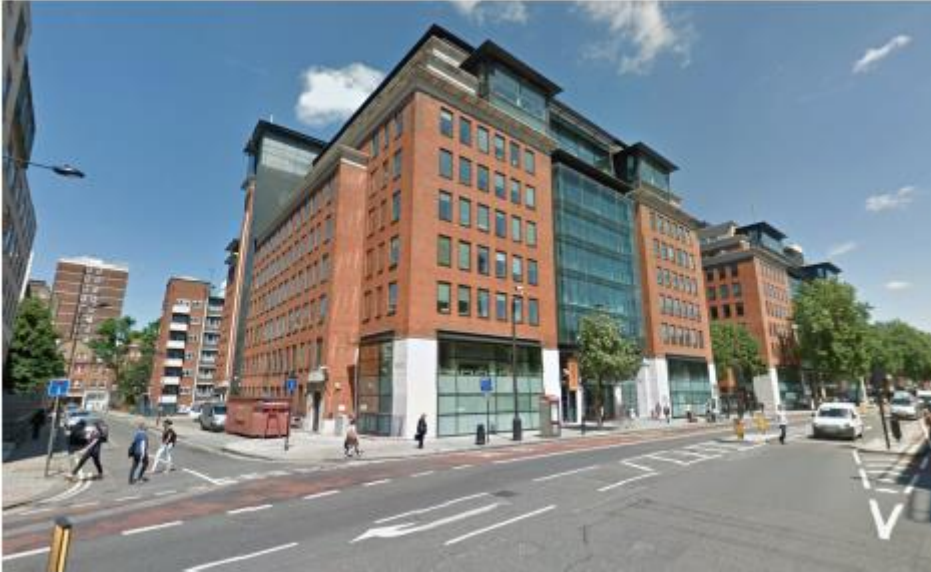
North West facing Photograph of existing Warner House
