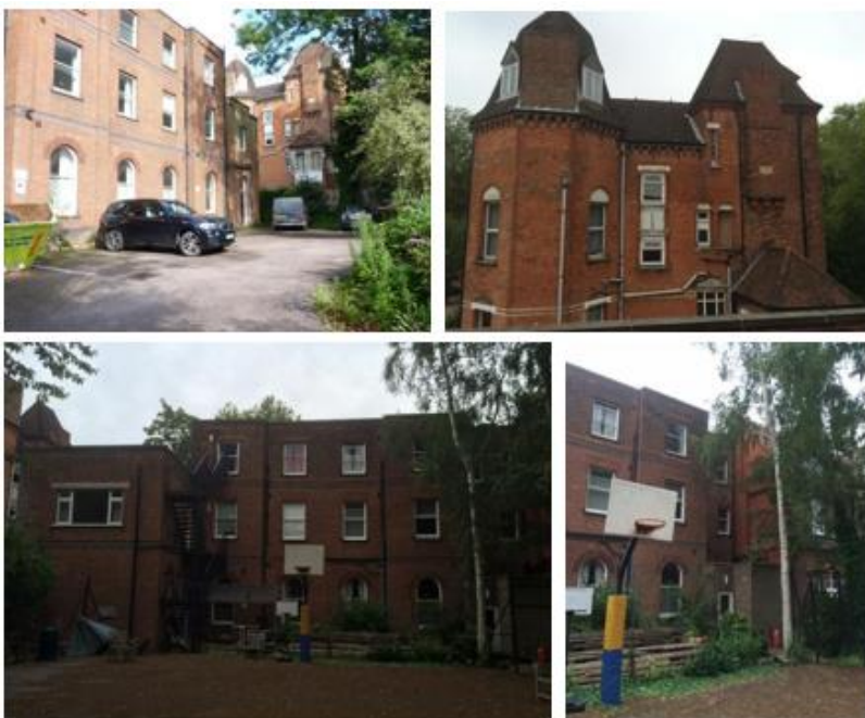
View of north-wing and of no.43
