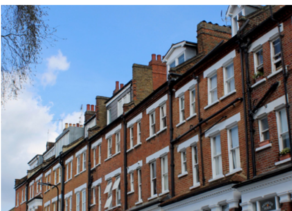
Variety of Front dormer windows
